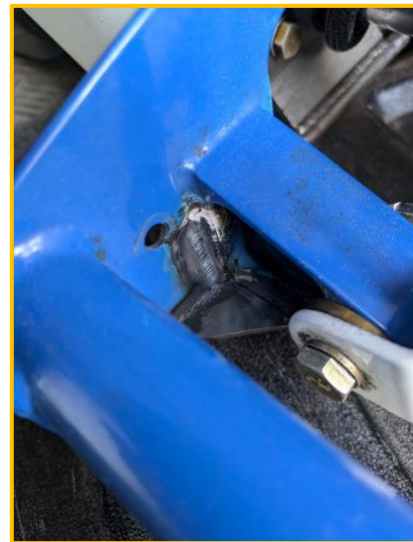
Original crack rewelded
